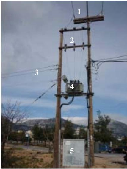
**Figure 1.** Typical configuration of a two-pole type distribution substation. 1:Medium Voltage Line, 2:Fuse Disconnectors, 3: Low Voltage Line, 4:Transformer, 5: Low Voltage switchgear.
